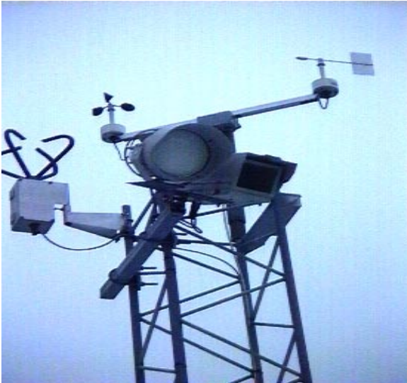
RWIS -site with sensors for wind-speed and wind-direction, the Optic-Eye for precipitation. Camera and Infrared floodlight for pictures.
